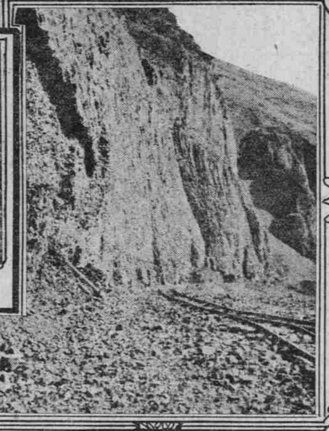
HEAVY WORK ON THE DESCHUTES RAILROAD NEAR SHEARER'S BRIDGE
