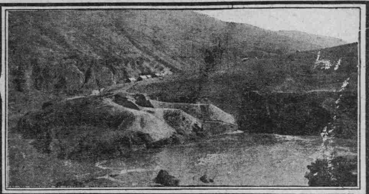
THREE CUTS AND FILLS MADE BY OREGON TRUNK LINE IN OVERCOMING DIFFICULT CONSTRUCTION AT THE OXBOW.
