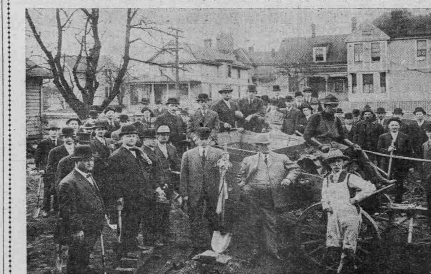
EXALTED RULER PADDEN, HOLDING SPADE WITH WHICH FIRST EARTH WAS REMOVED FROM EXCAVATION.
