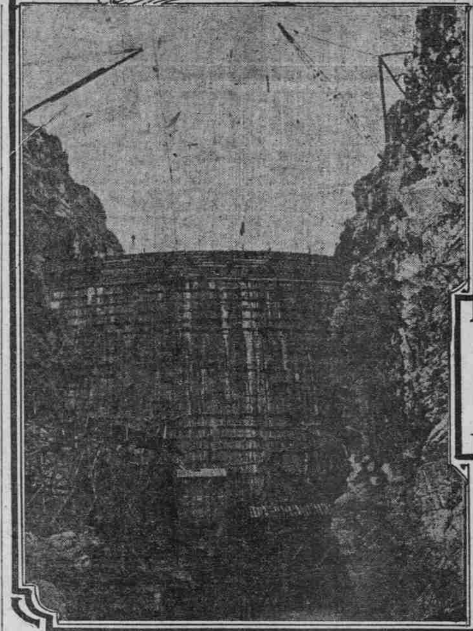
BUILDING THE CONCRETE AND ROCK BALLASTED SHOSHONE DAM, THE HIGHEST DAM IN THE WORLD.
