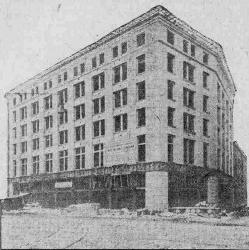
NEW STRUCTURE UNDER WAY FOR BLAKE McFALL COMPANY AT FOURTH AND ANKENY STREETS.
