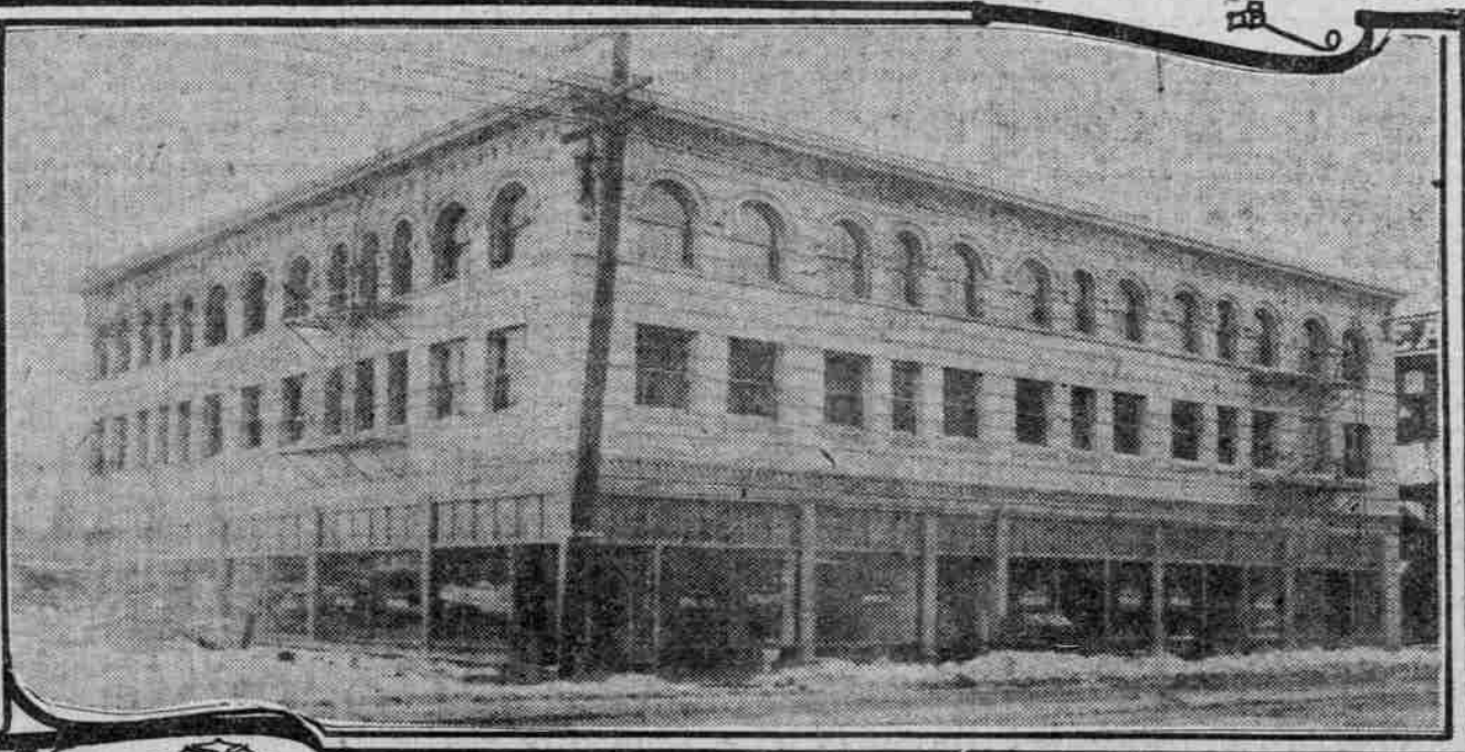
COOK AND LEITH BUILDING, E. STARK & GRAND AVES.
