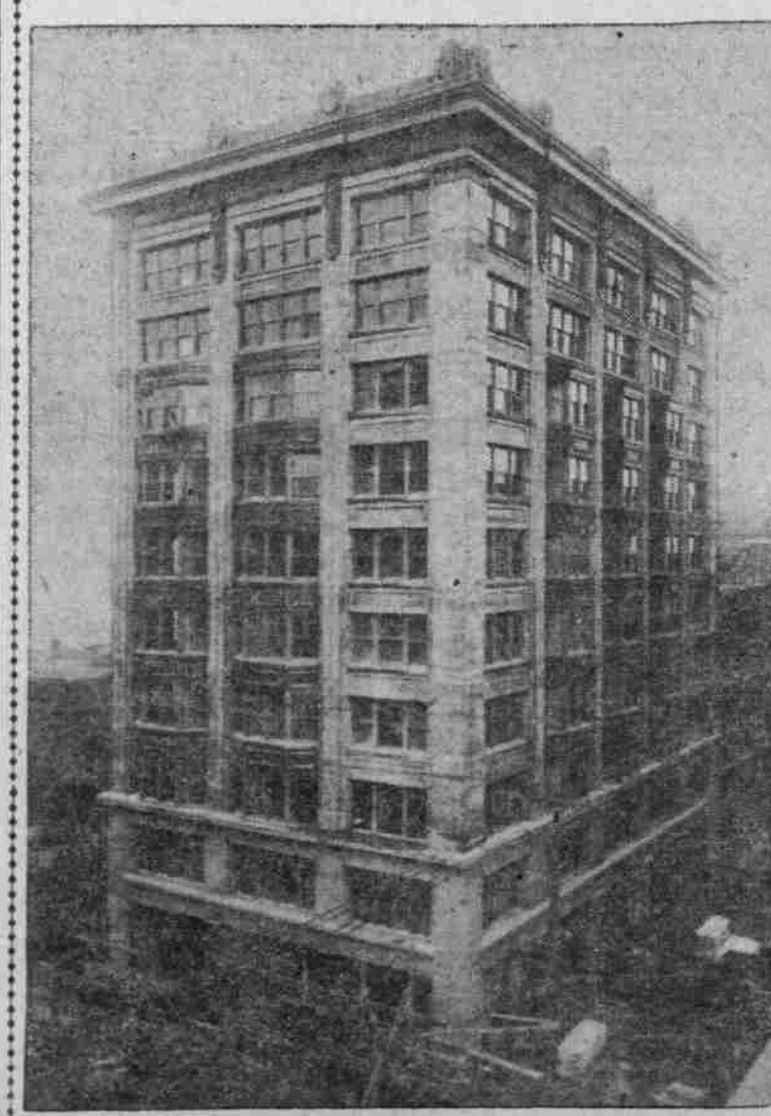
LEWIS BLOCK, UNDER CONSTRUCTION AT FOURTH AND OAK STS.
