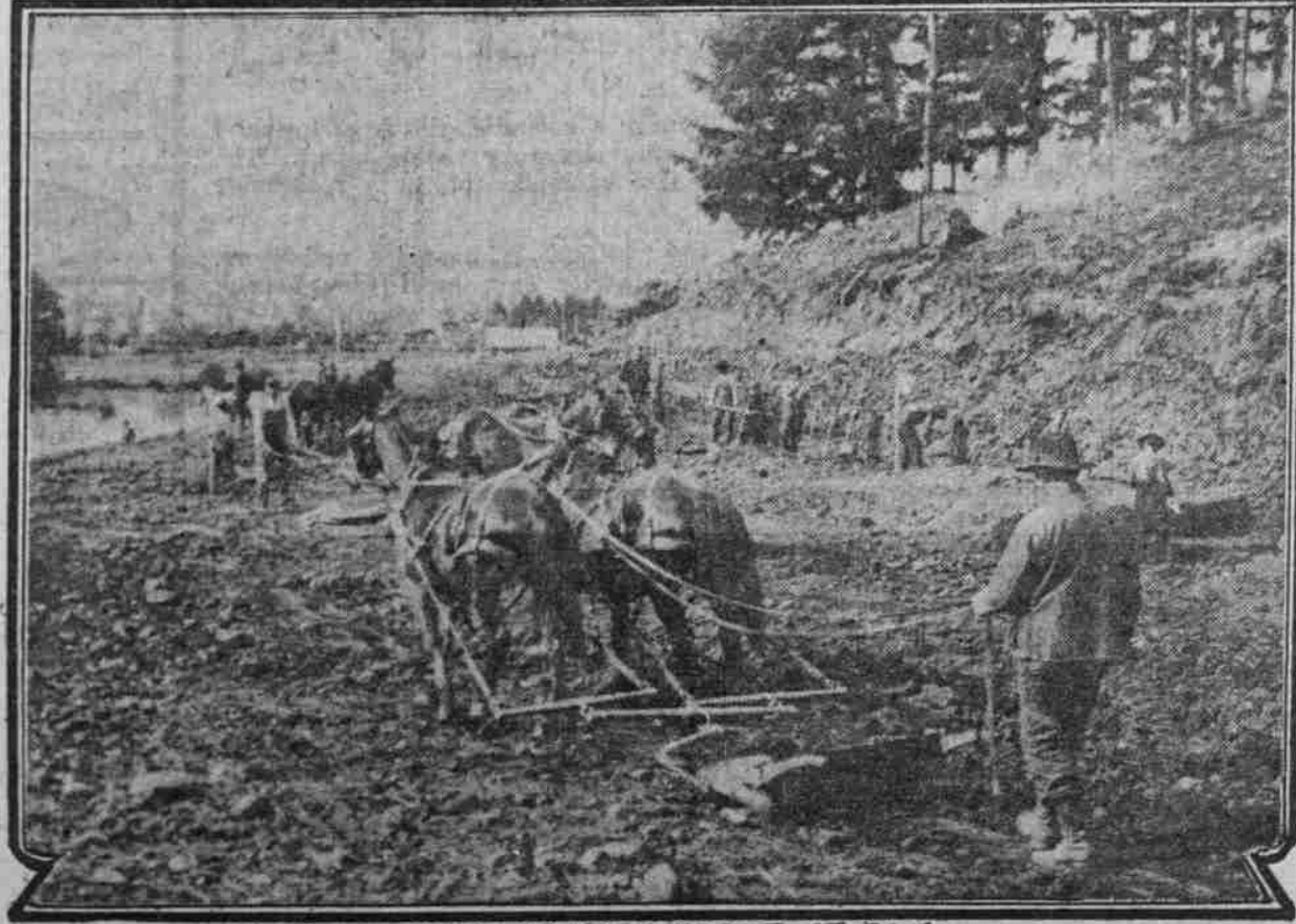
MEN AND TEAMS AT WORK ON SITE OF DAM
