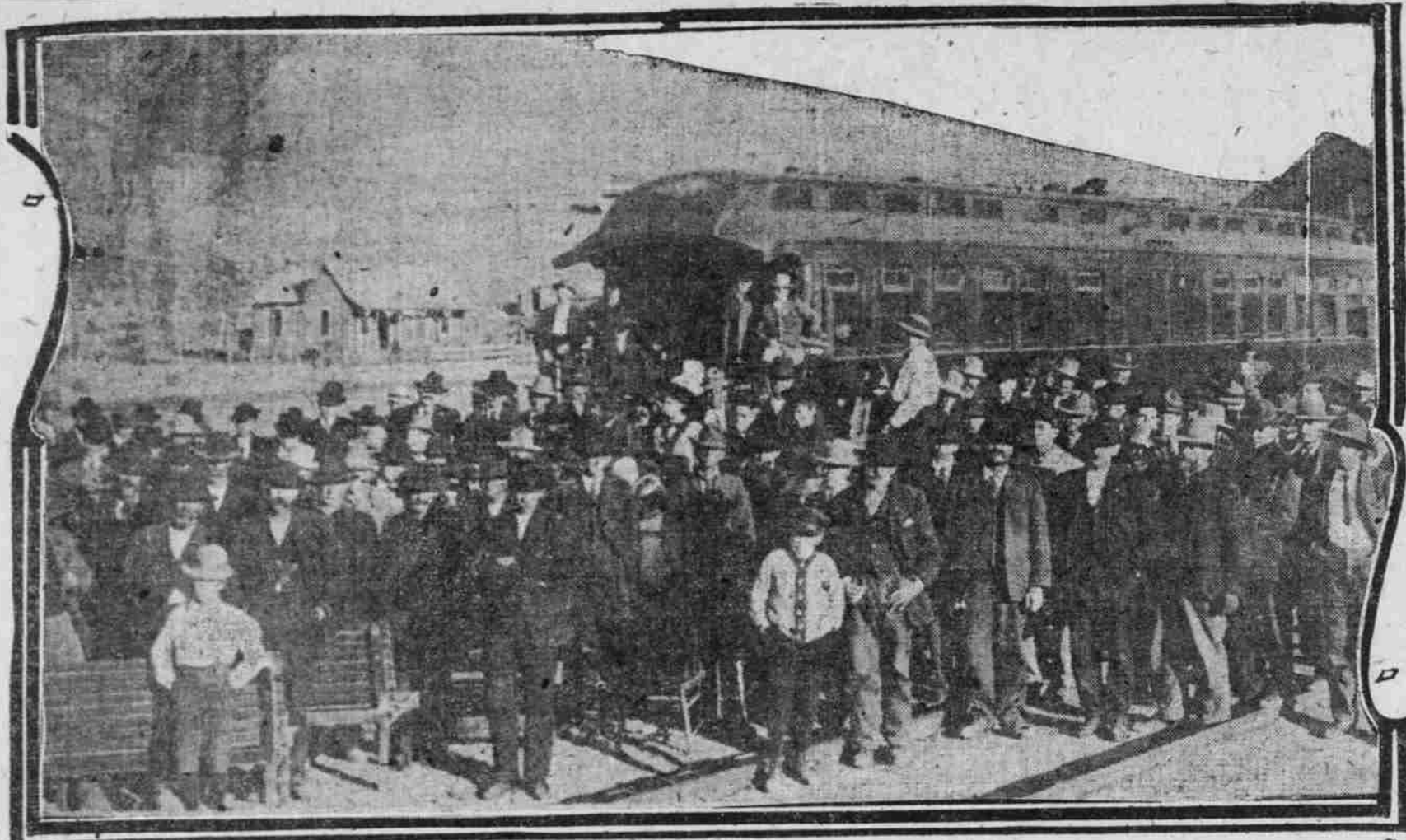
DEMONSTRATION TRAIN AT HEPPNER
