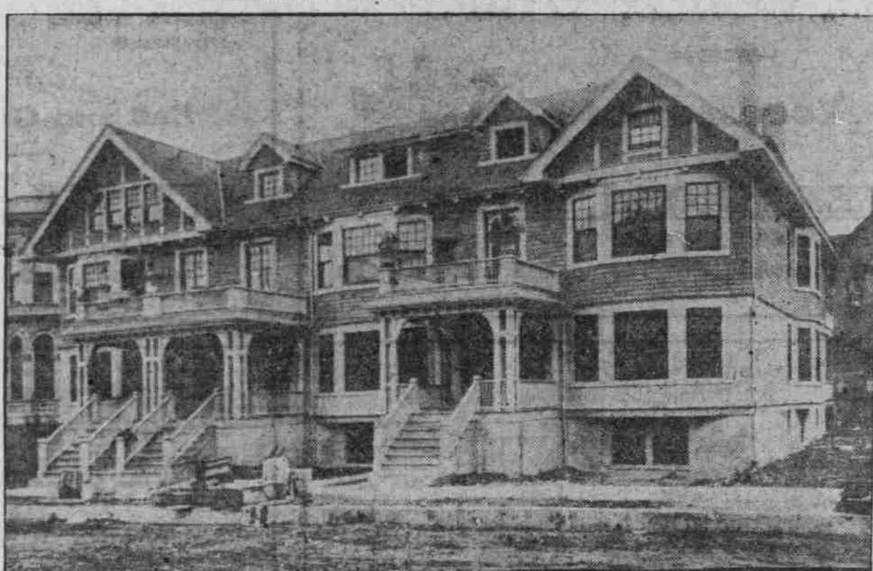
SIX-APARTMENT-HOUSE, COSTING $15,000 ON HOYT STREET, NEAR TWENTY-FIRST, BUILT FOR MRS. FLORENCE McDONNELL.
