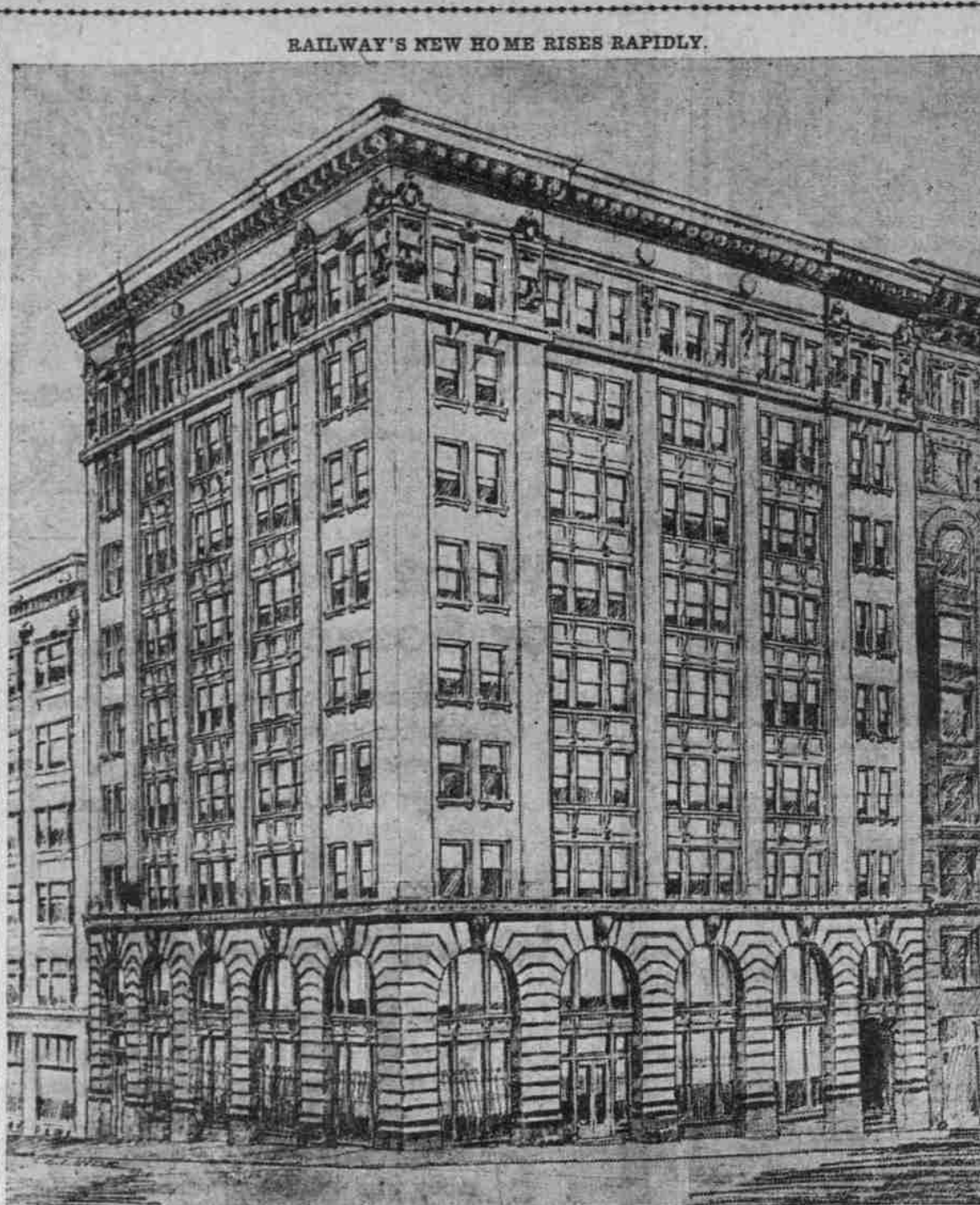
ELECTRIC BUILDING AT SEVENTH AND ALDER STREETS AS IT WILL APPEAR WHEN COMPLETED.
