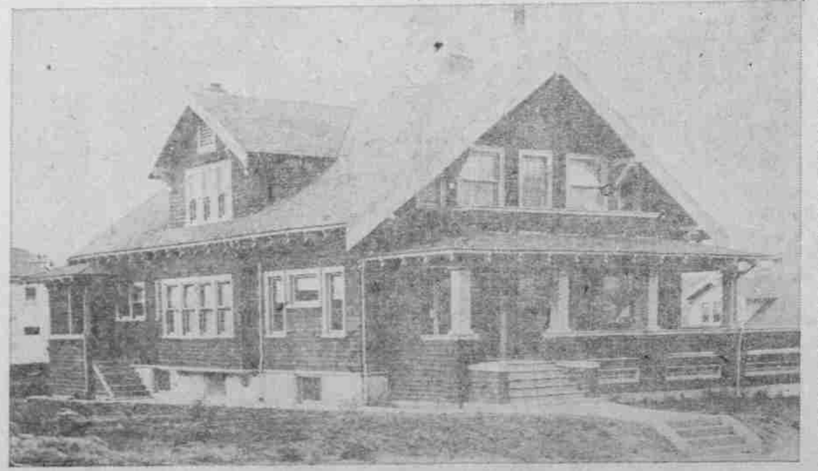
THE $6000 SWISS CHALET BUNGALOW HOME OF D. R. FLICKINGER, CORNER OF EAST SEVENTY-FIRST AND YAMHILL STREETS, JUST COMPLETED.
