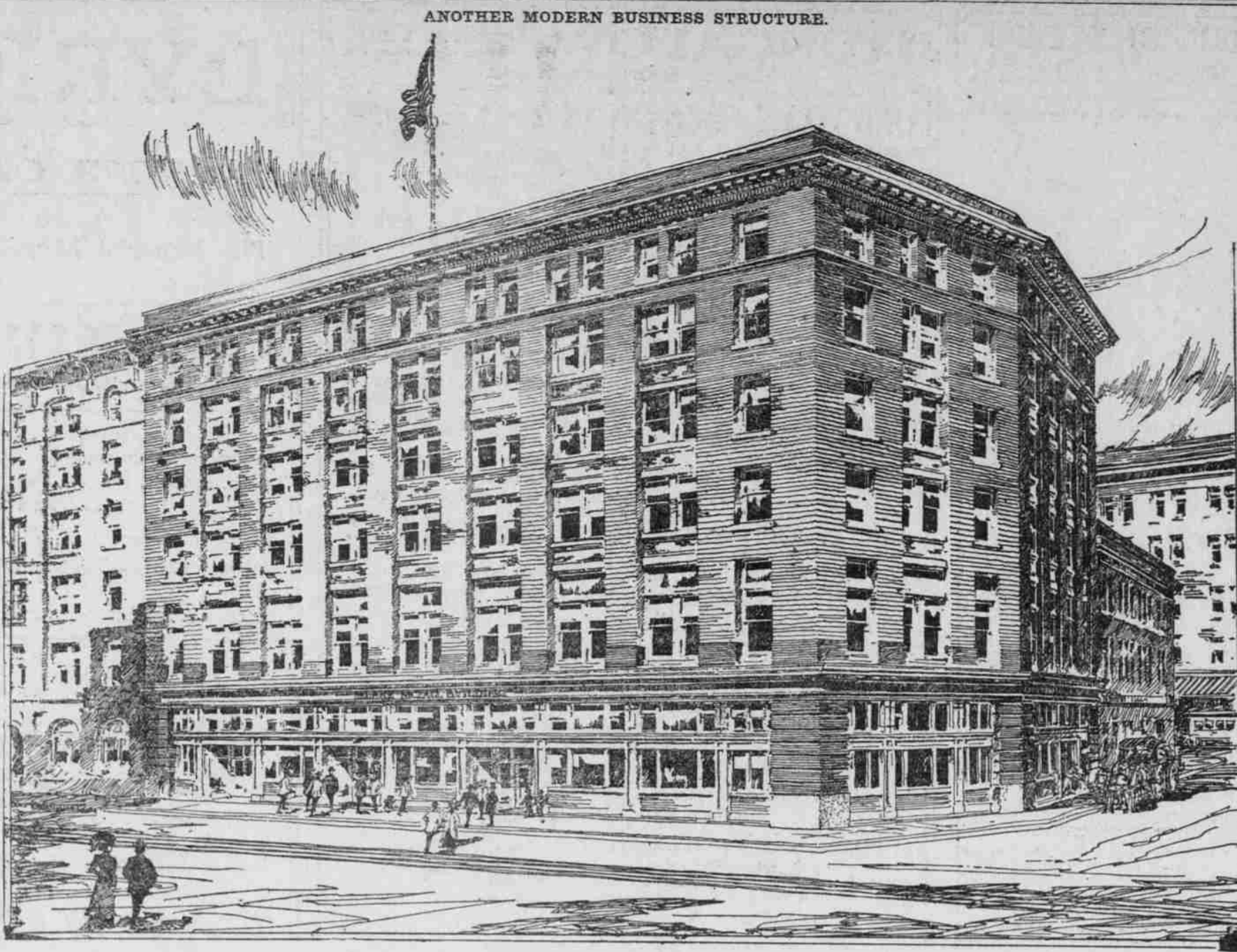
BLAKE, McFALL BUILDING TO BE ERRECTED AT FOURTH AND ANKENY.
