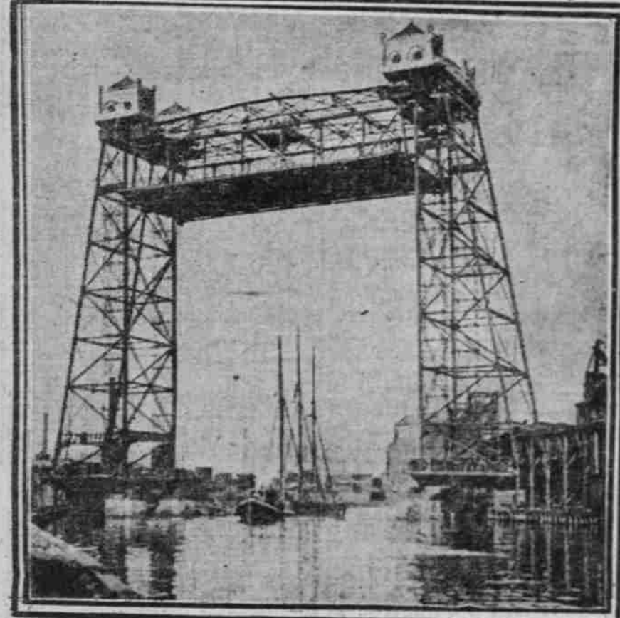
GENERAL VIEW OF HALSTED ST. LIFT BRIDGE OF CHICAGO WHEN SPAN IS LIFTED CLEAR UP. THIS SPAN CAN BE RAISED TO ENTIRE HEIGHT OF 140 FT. IN 34 SECONDS.
