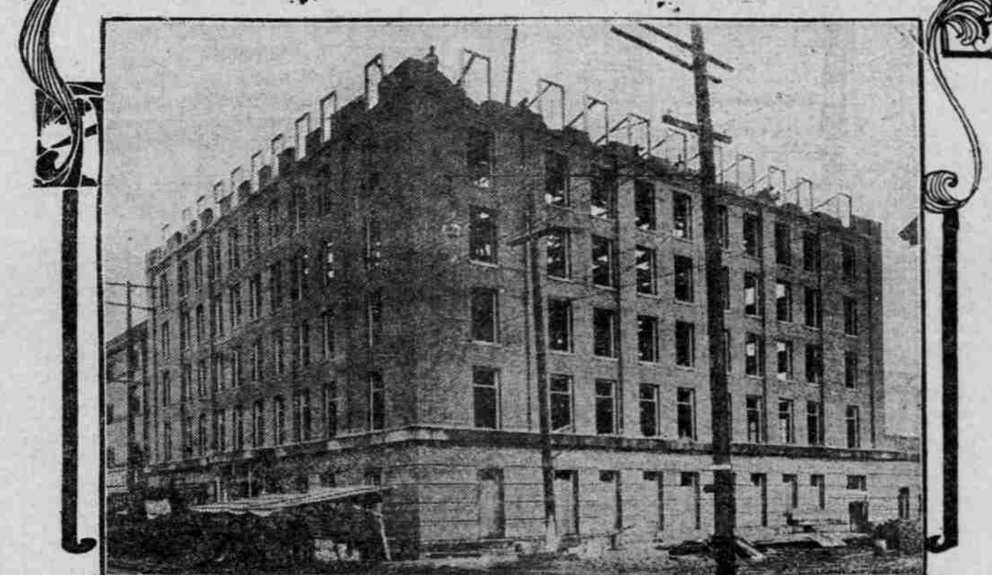
CRANE WAREHOUSE, 14TH AND IRVING
