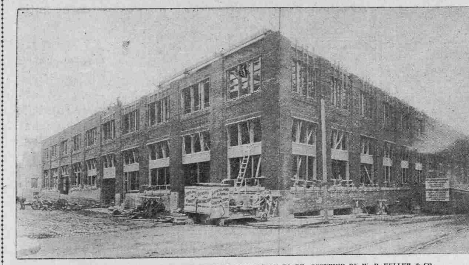
CONCRETE AND BRICK BUILDING NEARING COMPLETION TO BE OCCUPIED BY W. P. FULLER & CO.
