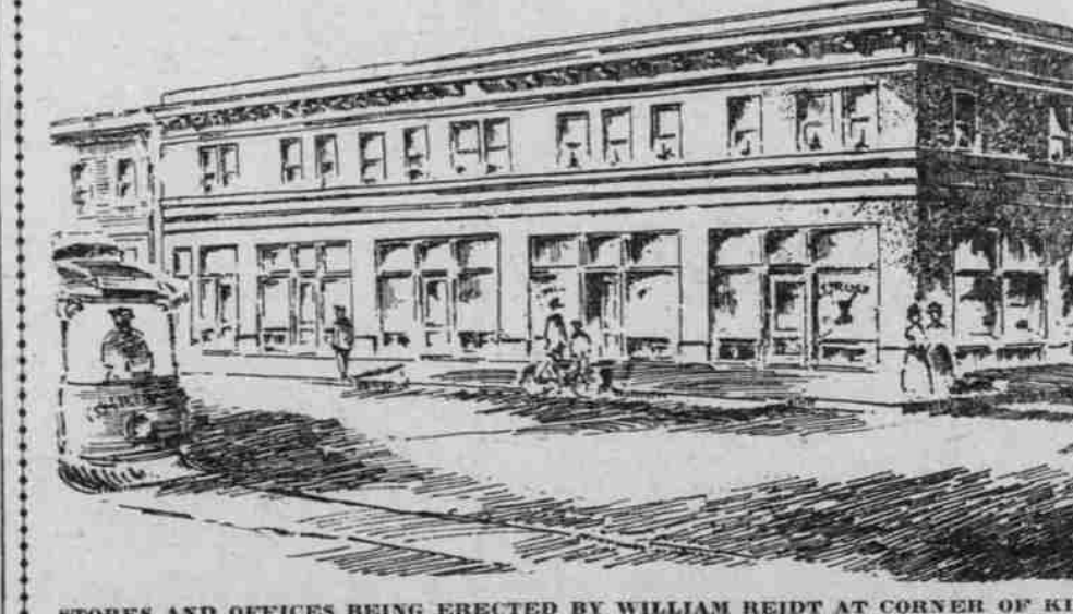
STORES AND OFFICES BEING ERRECTED BY WILLIAM REID AT CORNER OF KILLINGSWORTH AVENUE.
