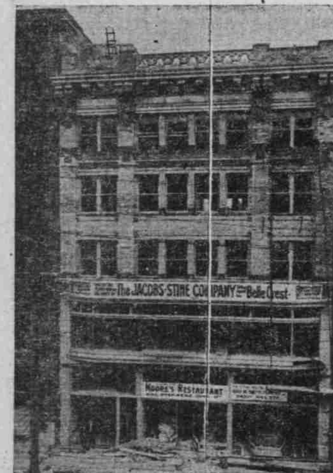
This Looks Good, the Entire Fifth Floor Is the Factory, 2 Elevators
