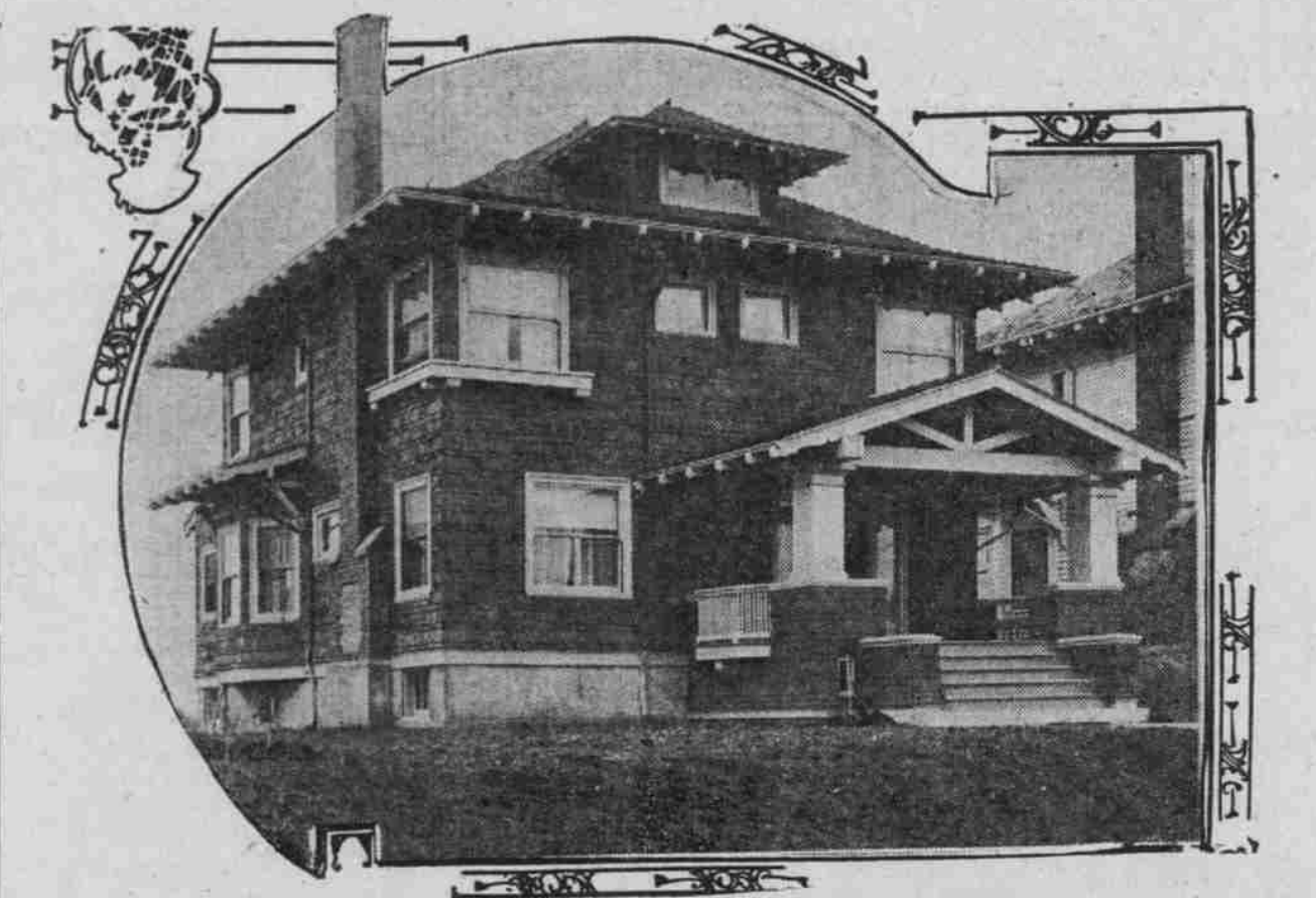
NEW RESIDENCE OF J. S. GREENY, 295 EAST TWENTY-THIRD STREET.
