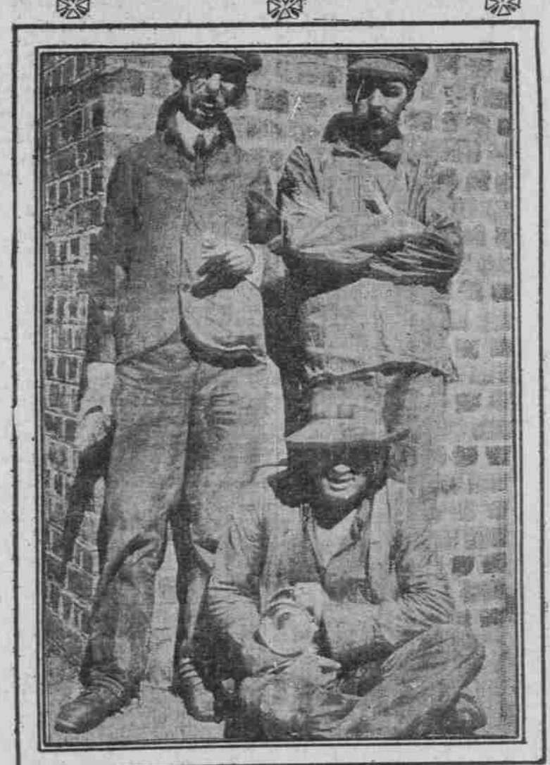
"READY FOR THE UNDERGROUND," MAN AT RIGHT IS AMERICAN MANAGER, MR. CARPENTER AT LEFT
