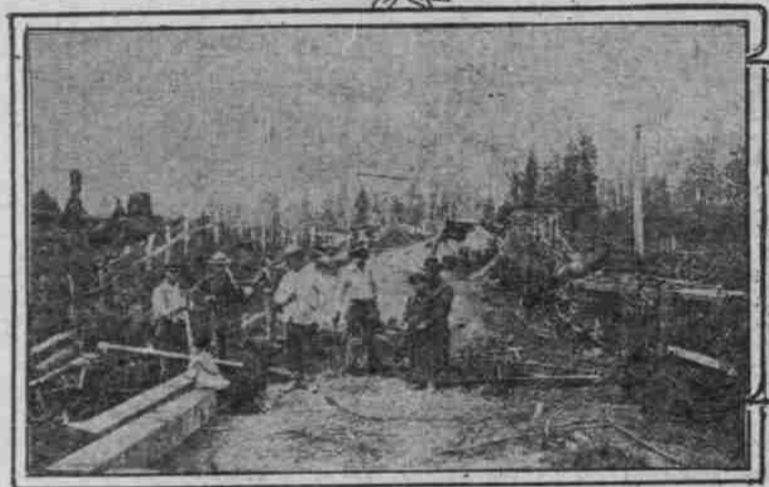
RECONSTRUCTING AN OLD ROAD
