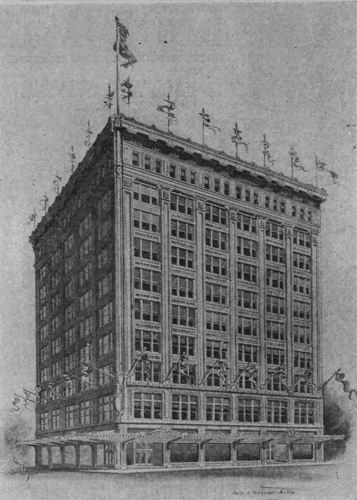
HANDSOME BUSINESS BUILDING, AT SIXTH AND ALDER STREETS, WILL BE RUSHED TO COMPLETION.
