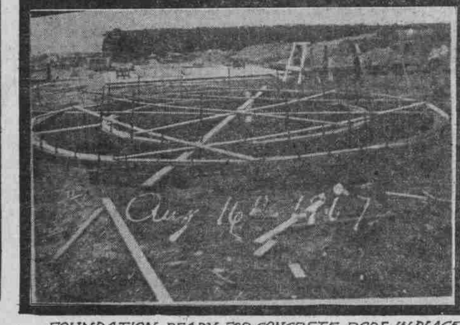
FOUNDATION READY FOR CONCRETE, RODS IN PLACE. POINT ARENA LIGHT STATION.
