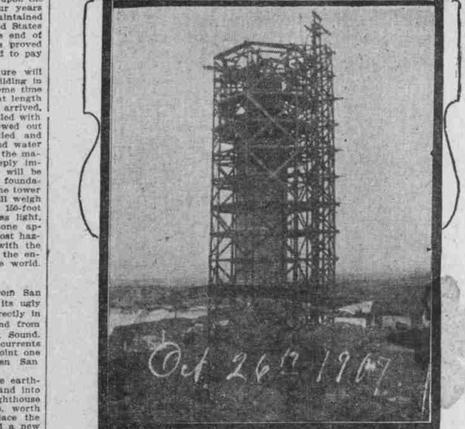
POINT ARENA - TOWER IN COURSE OF CONSTRUCTION, SHOWING STAGING.
