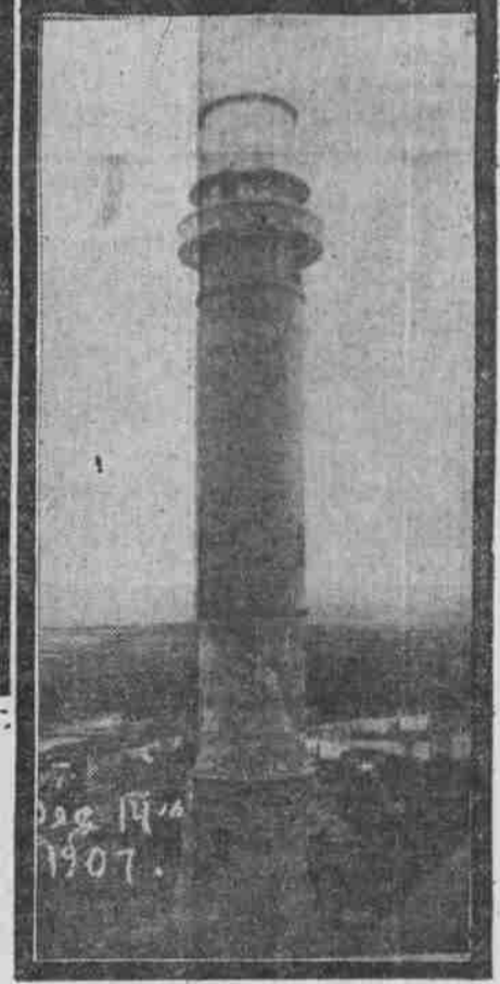
POINT ARENA LIGHTHOUSE COMPLETED. FIRST REINFORCED CONCRETE LIGHTHOUSE IN AMERICA!
