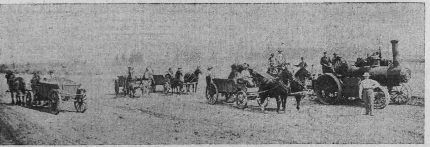
The accompanying illustration shows how Elwood Wiles is improving and grading the streets in what was known as the old Irvington, race track. This grading outfit is the most improved and up-to-date in the city.
