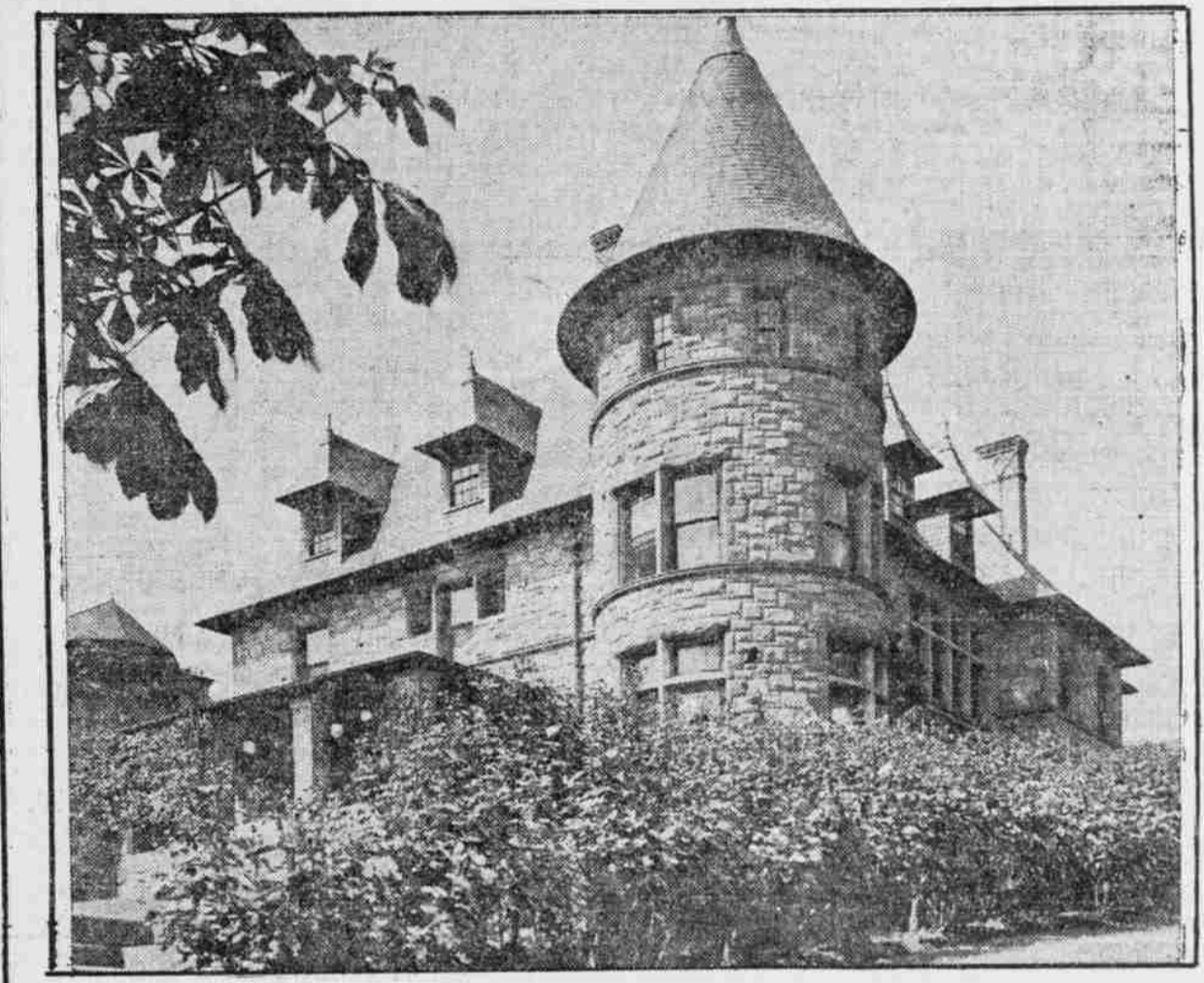
RESIDENCE OF DAVID J. HONEYMAN, 193 KING ST.
