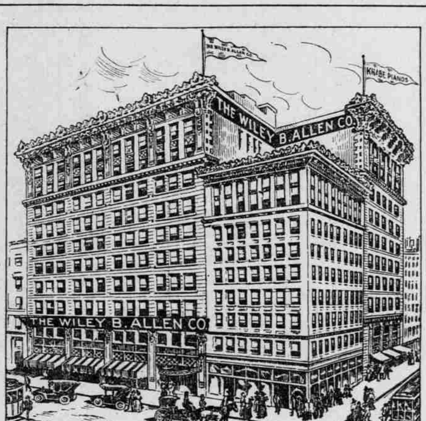
The new headquarters of the Wiley B. Allen Co. now under way of construction at the corner of Kearny and Sutter streets, San Francisco, one of the largest establishments in the world devoted exclusively to the sale of pianos.
