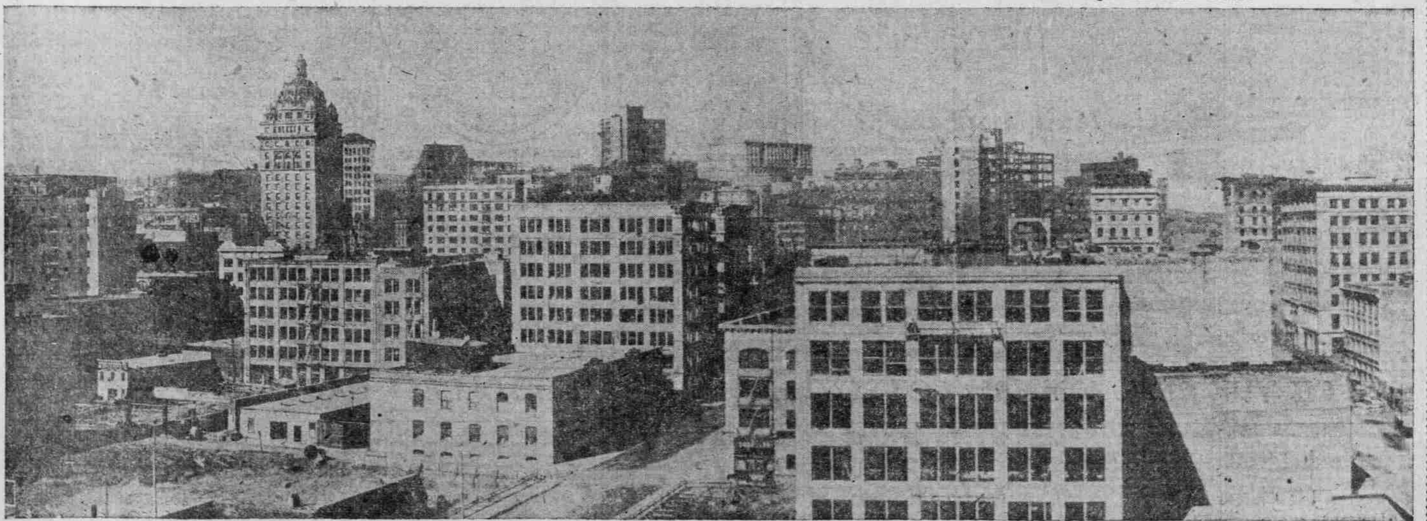
RECENT PHOTOGRAPHIC VIEW OF COAST METROPOLIS, SHOWING PROGRESS MADE IN REBUILDING.
