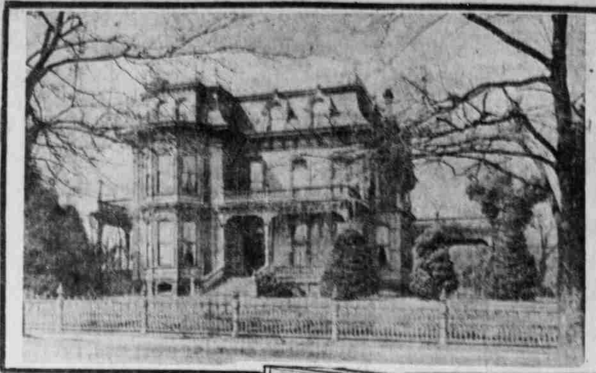
TAILING RESIDENCE 5TH AND SALMON STS.
