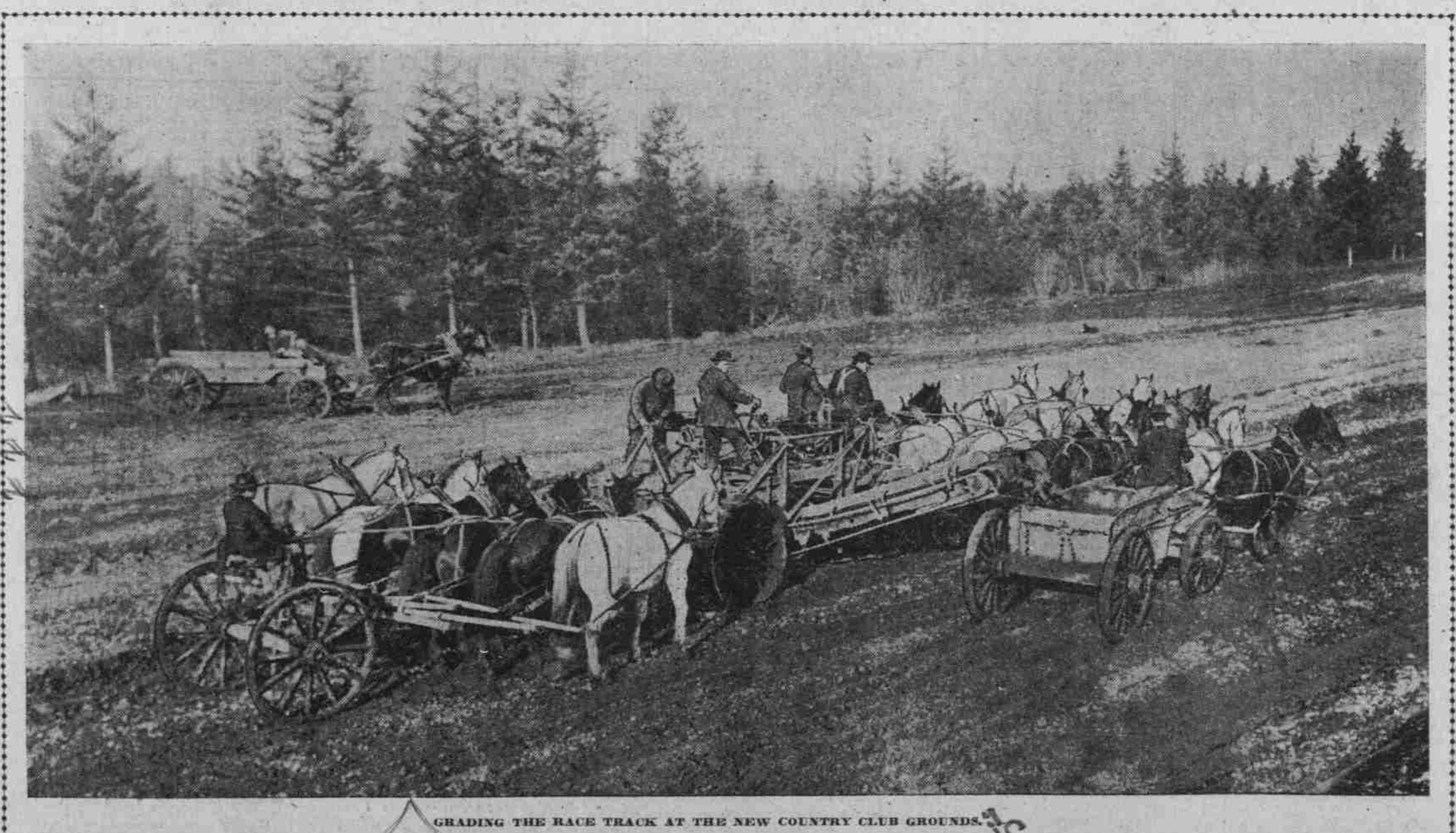
GRADING THE RACE TRACK AT THE NEW COUNTRY CLUB GROUNDS.
