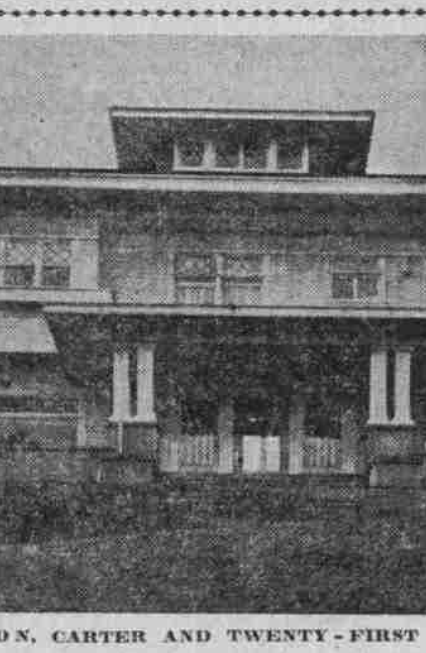
RESIDENCE OF E. L. THOMPSON, CARTER AND TWENTY-FIRST STREETS, PORTLAND HEIGHTS
