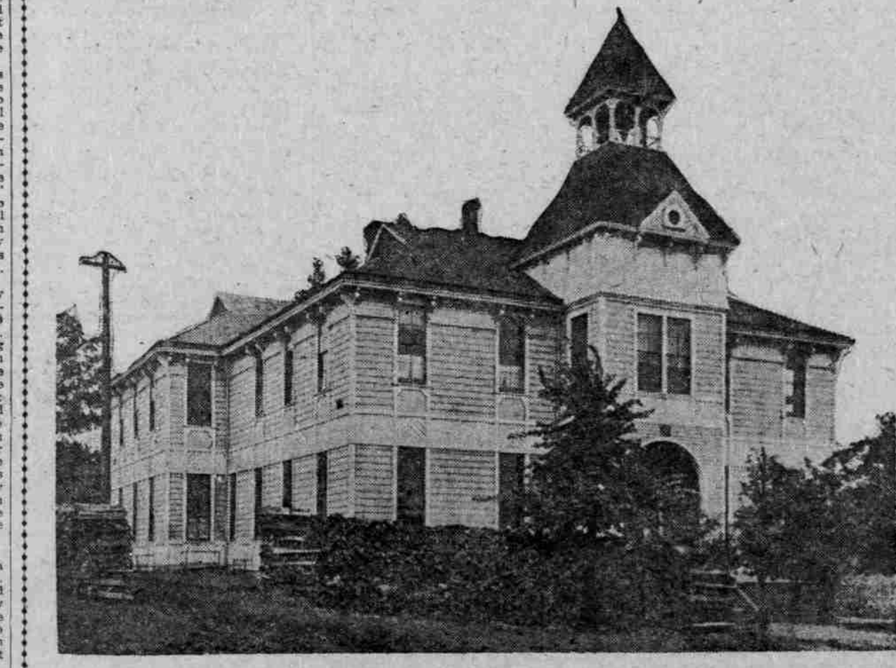
PRESENT STRUCTURE IS ONE OF THE OLDEST IN THE CITY.
