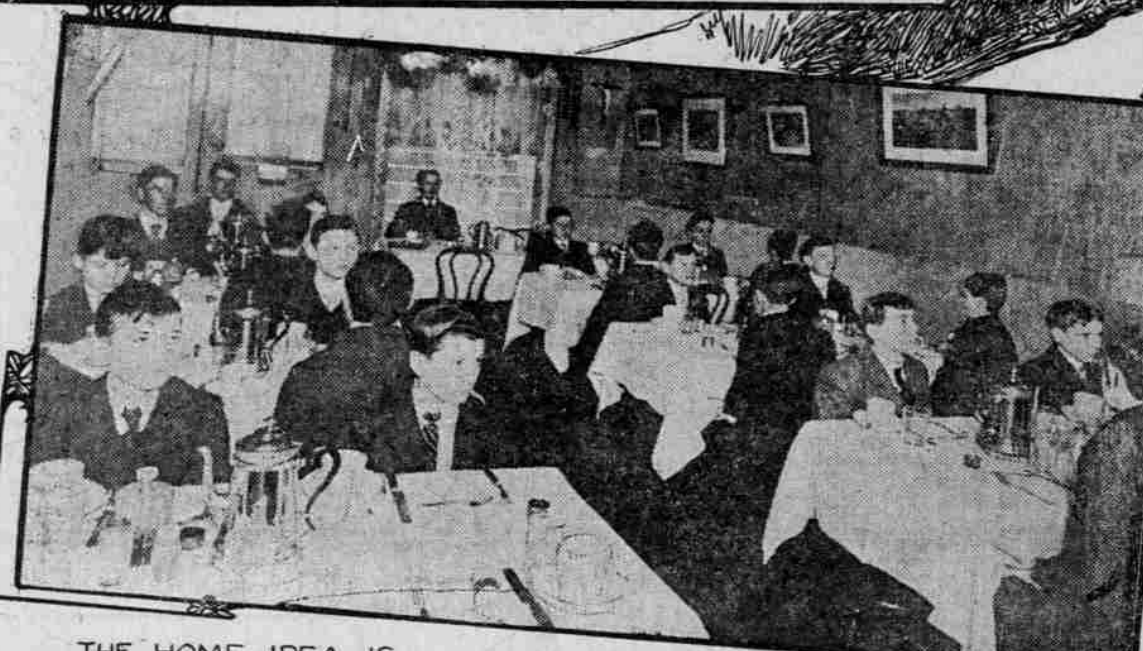
THE HOME IDEA IS EFFECTIVELY EXPRESSED IN THE DINING ROOM.
