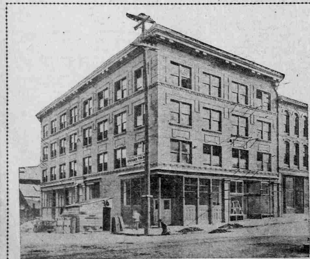
MEAD ESTATE BUILDING BEING COMPLETED AT FIRST AND COLUMBIA STREETS.
