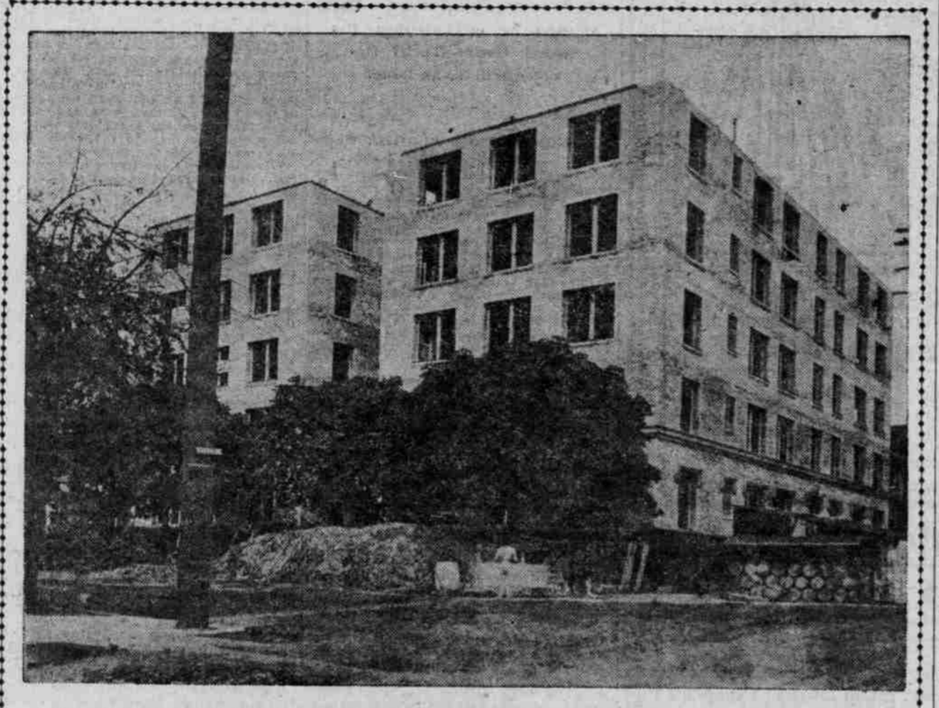
SEVEN-STORY HOTEL BEING ERECTED FOR R. B. LAMSON AT ELEVENTH AND STARK STREETS.
