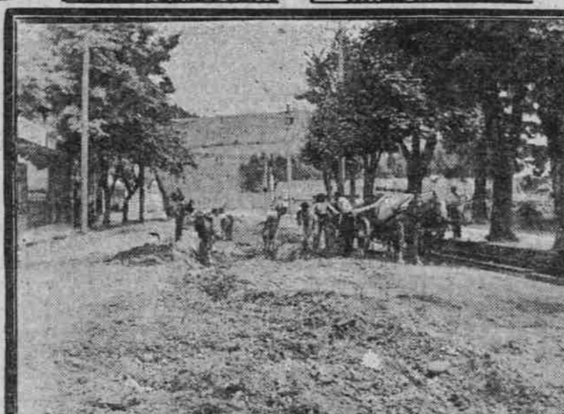
EXCAVATING FOR THE RAILWAY TRACK
