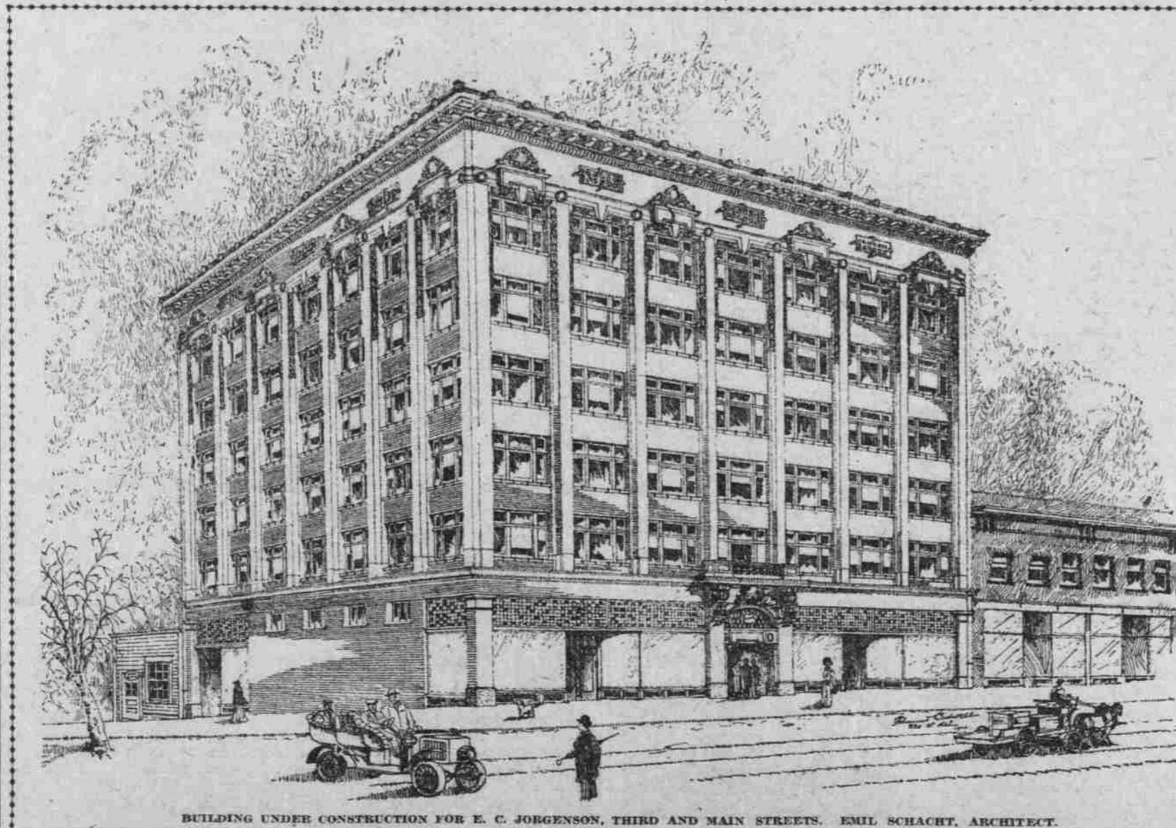
BUILDING UNDER CONSTRUCTION FOR E. C. JORGENSEN, THIRD AND MAIN STREETS. EMUL SCHACHT, ARCHITECT.
