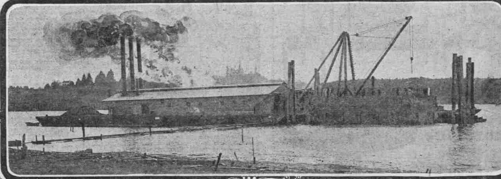
WHERE THE AIR COMPRESSORS ARE HOUSED
