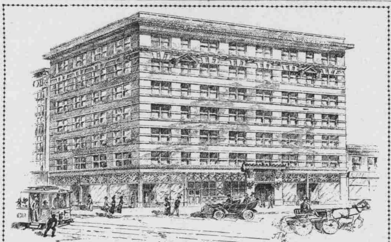
BRICK BUILDING NOW UNDER CONSTRUCTION FOR L. Q. SWETLAND, FIFTH AND WASHINGTON STREETS. EMIL SCHACHT, ARCHITECT.
