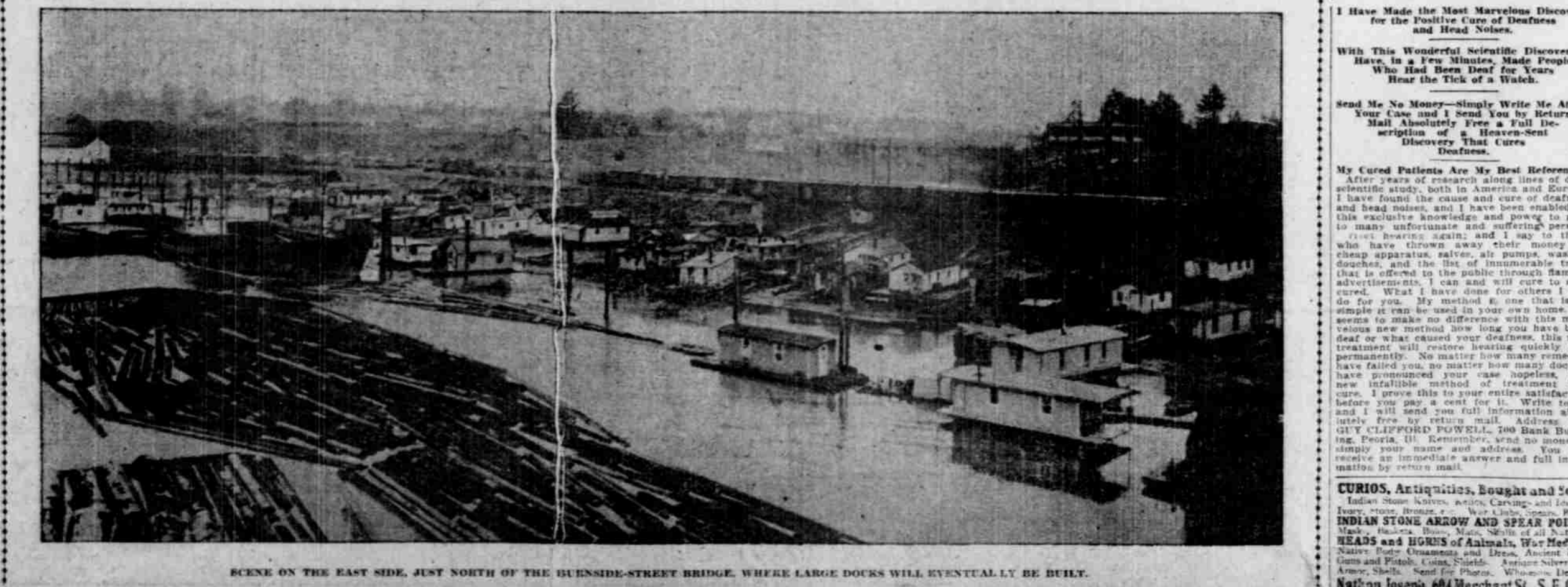
SCENE ON THE EAST SIDE, JUST NORTH OF THE GUARDSIDE-STREET BRIDGE, WHERE LARGE DOCKS WILL, EVENTUALLY, BE BUILT.
