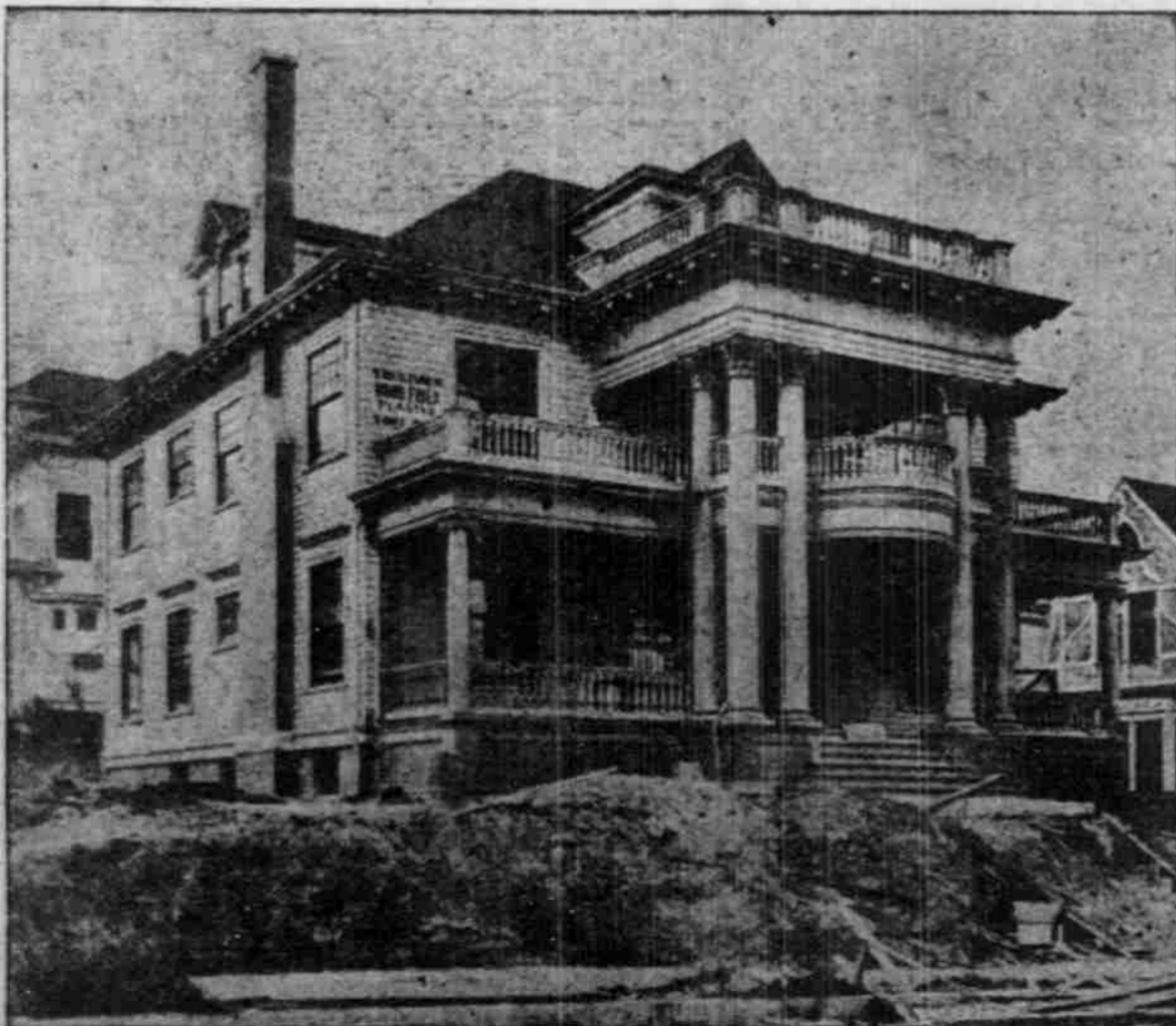
NEARING COMPLETION AT TWENTY-FOURTH AND KEARNEY STREETS.
