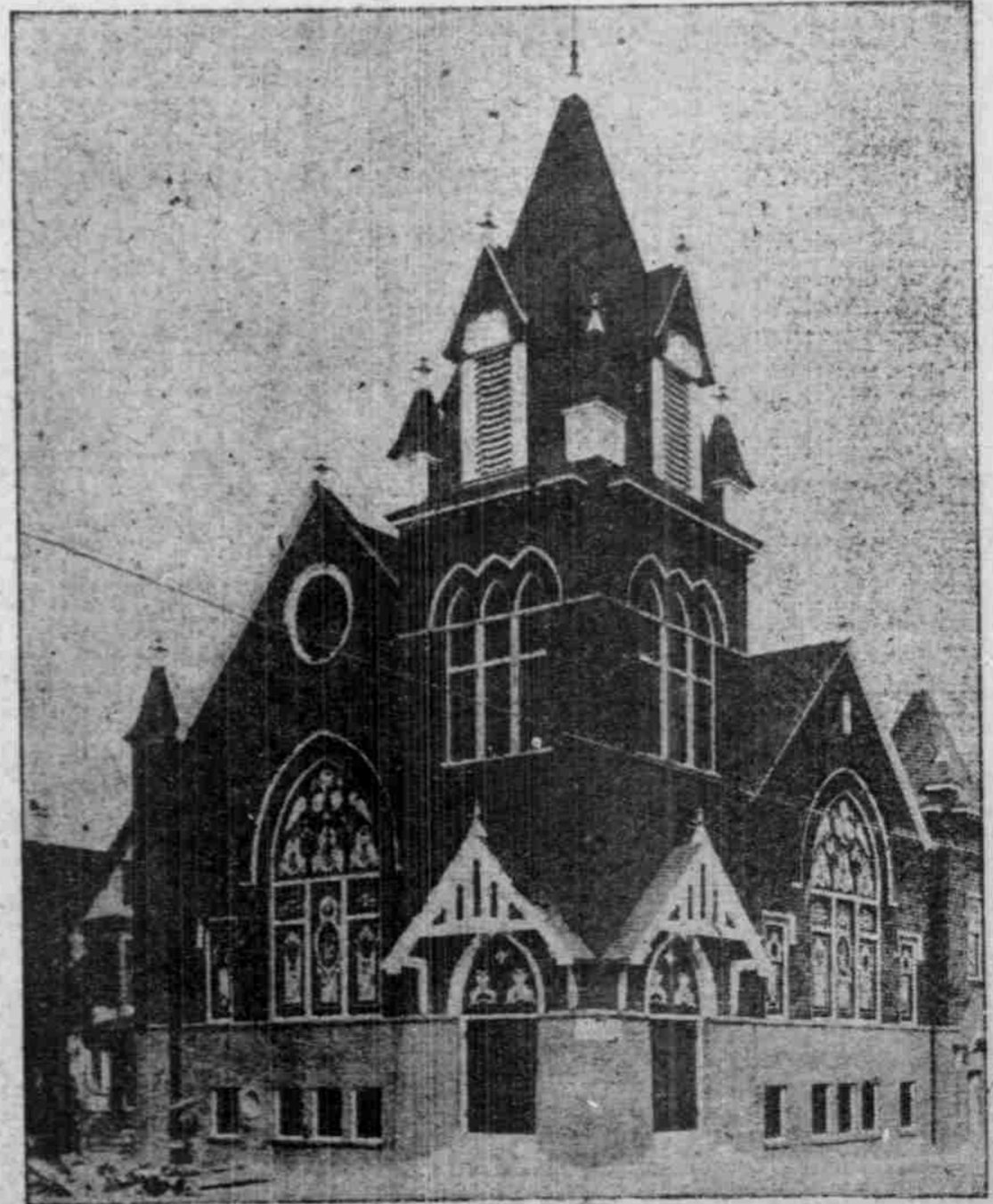
EDIFICE ERRECTED AT TENTH AND CLAY STREETS AT COST OF $11,000.
