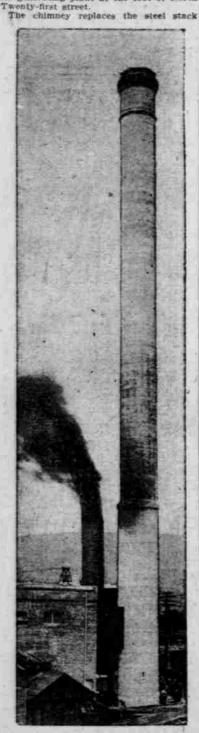
and induced system of draft heretofore in use and means a decided economy in the operation of the plant. This chimney is built of concrete, re-
