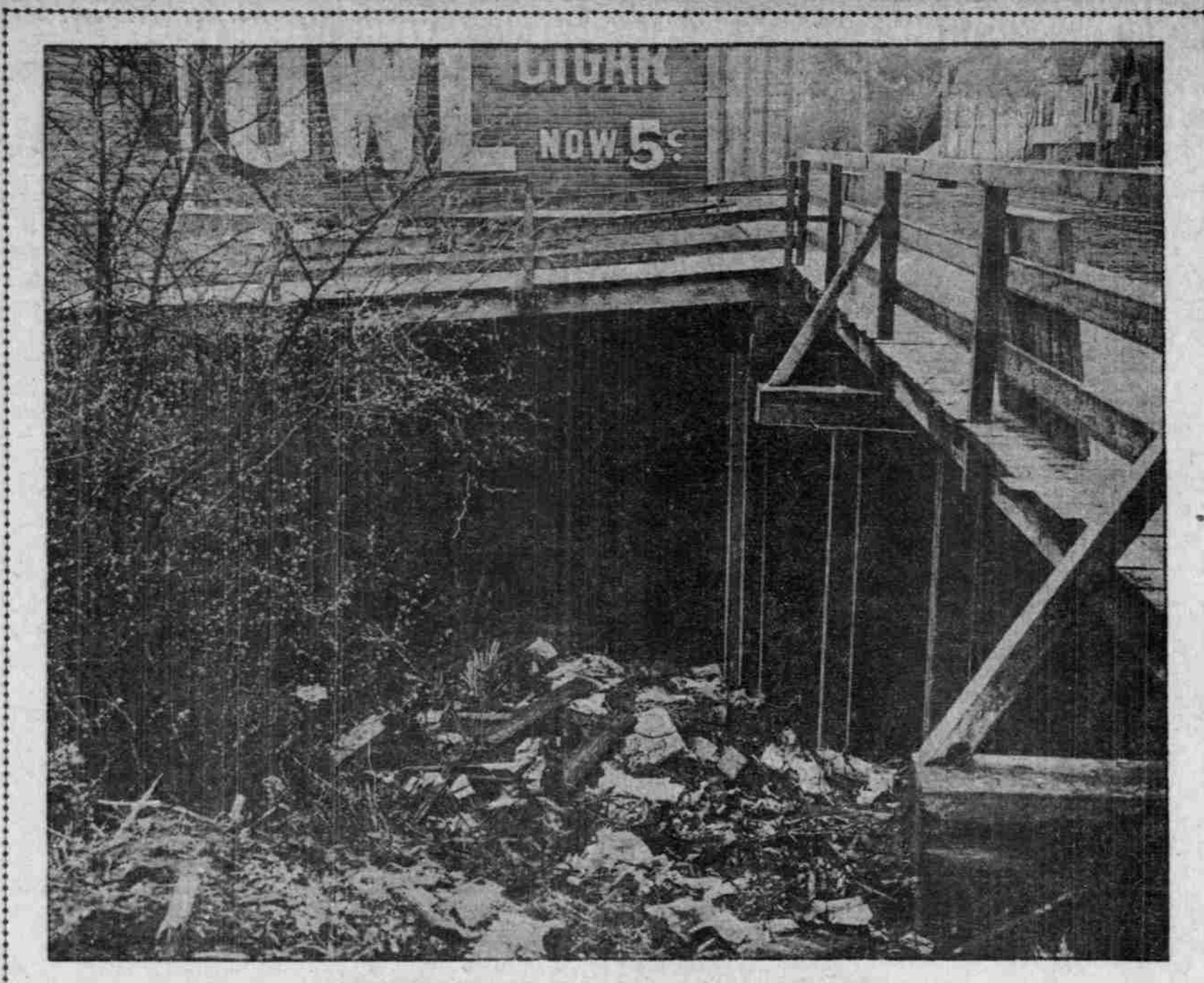
GARBAGE HEAP AT CORNER WILLIAMS AVENUE AND WEIDLER STREET.
