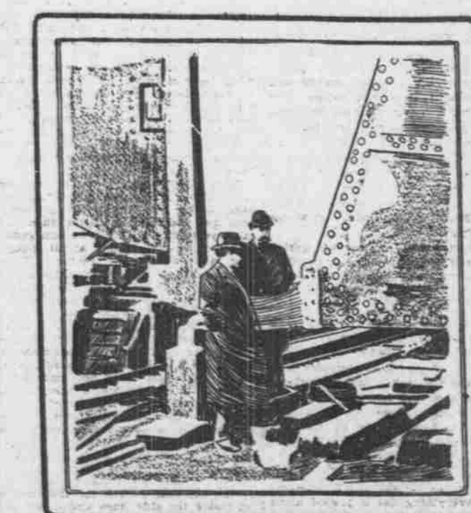
Stern post of the S. S. Sevilla (Hamburg American Line) welded in dry dock.
