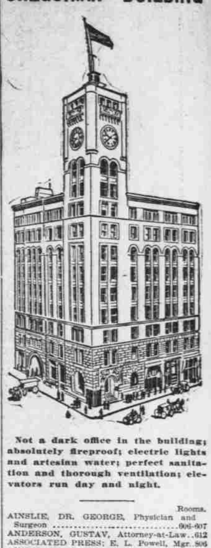
Not a dark office in the building; absolutely fireproof; electric lights and artesian water; perfect sanitation and thorough ventilation; elevators run day and night.
