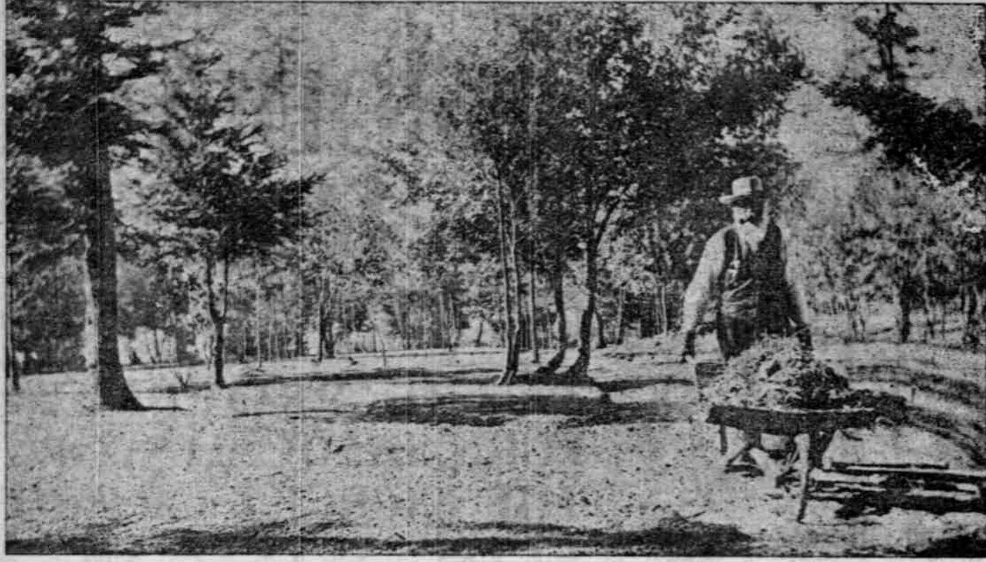
CLEANING THE GROUNDS IN PREPARATION TO SOWING GRASS SEED.
