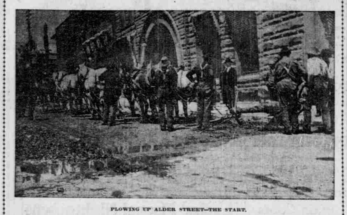
PLOWING UP ALDER STREET—THE START.
