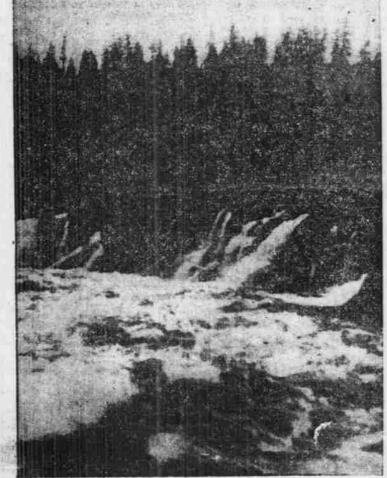
A sluice-way that affords an outlet into the river below the falls for the waste waters of the canal and looks that serve the dual purpose of floating the heavy river tonnage around Willamette Falls at Oregon City, and of furnishing power for running the large pulp and paper mills and other large manufacturing plants located at this site
