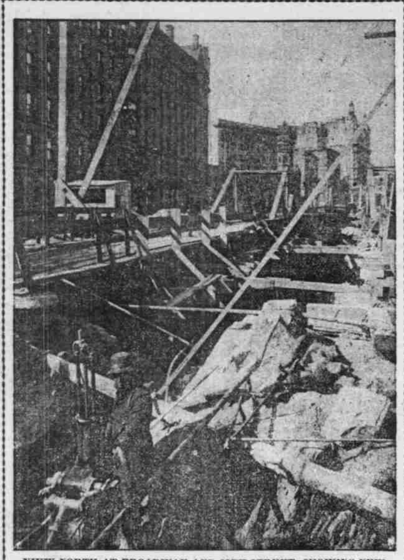
VIEW NORTH AT BROADWAY AND 69TH STREET—SHOWING ANSONIA HOTEL.
