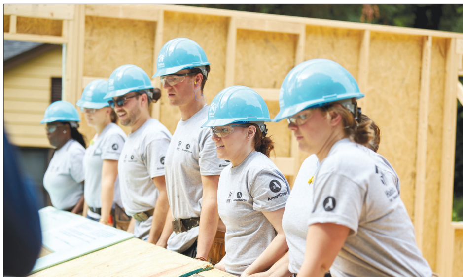
Habitat for Humanity, Portland Region
