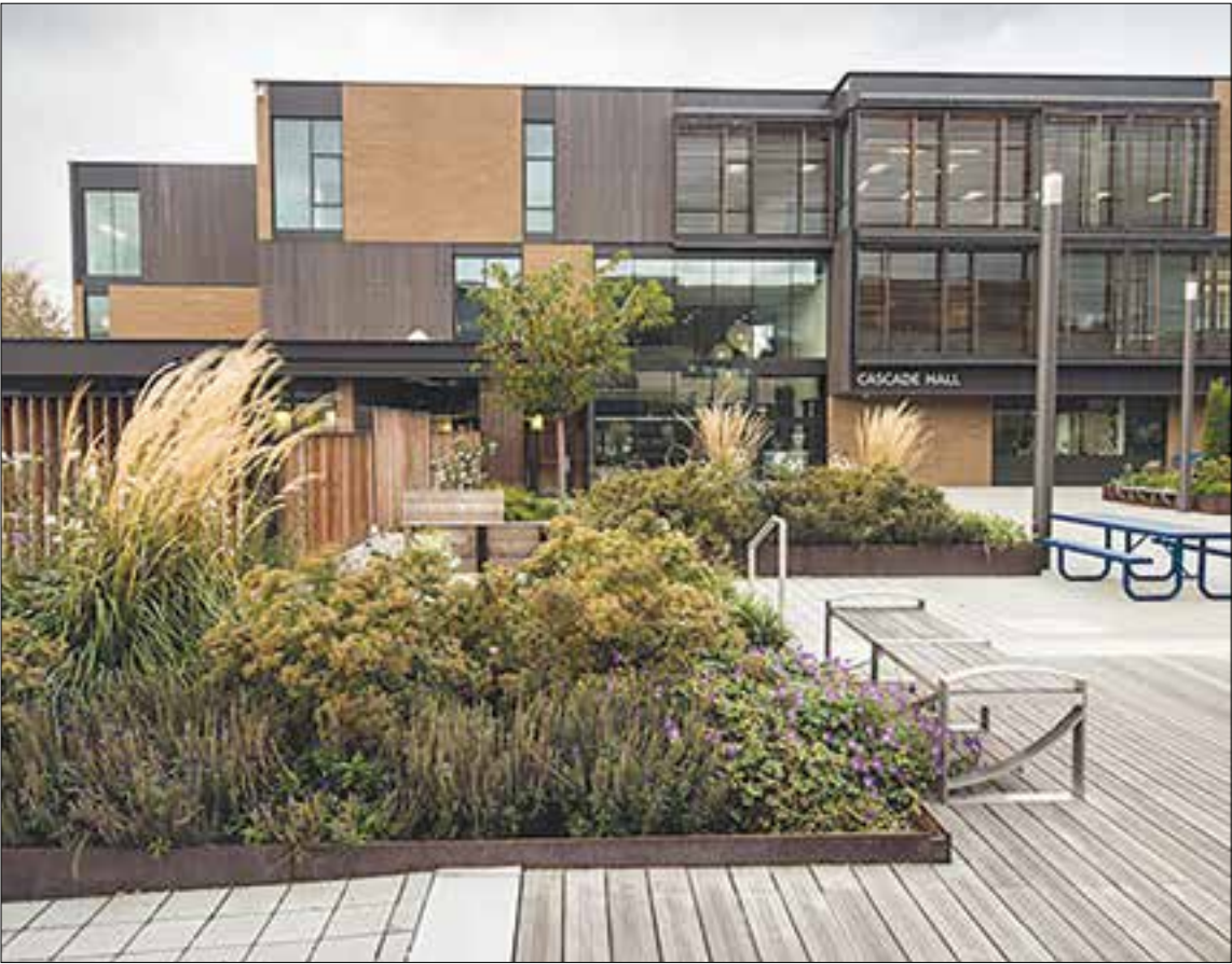
The PCC Cascade Hall. Photo Courtesy of Portland Community College
