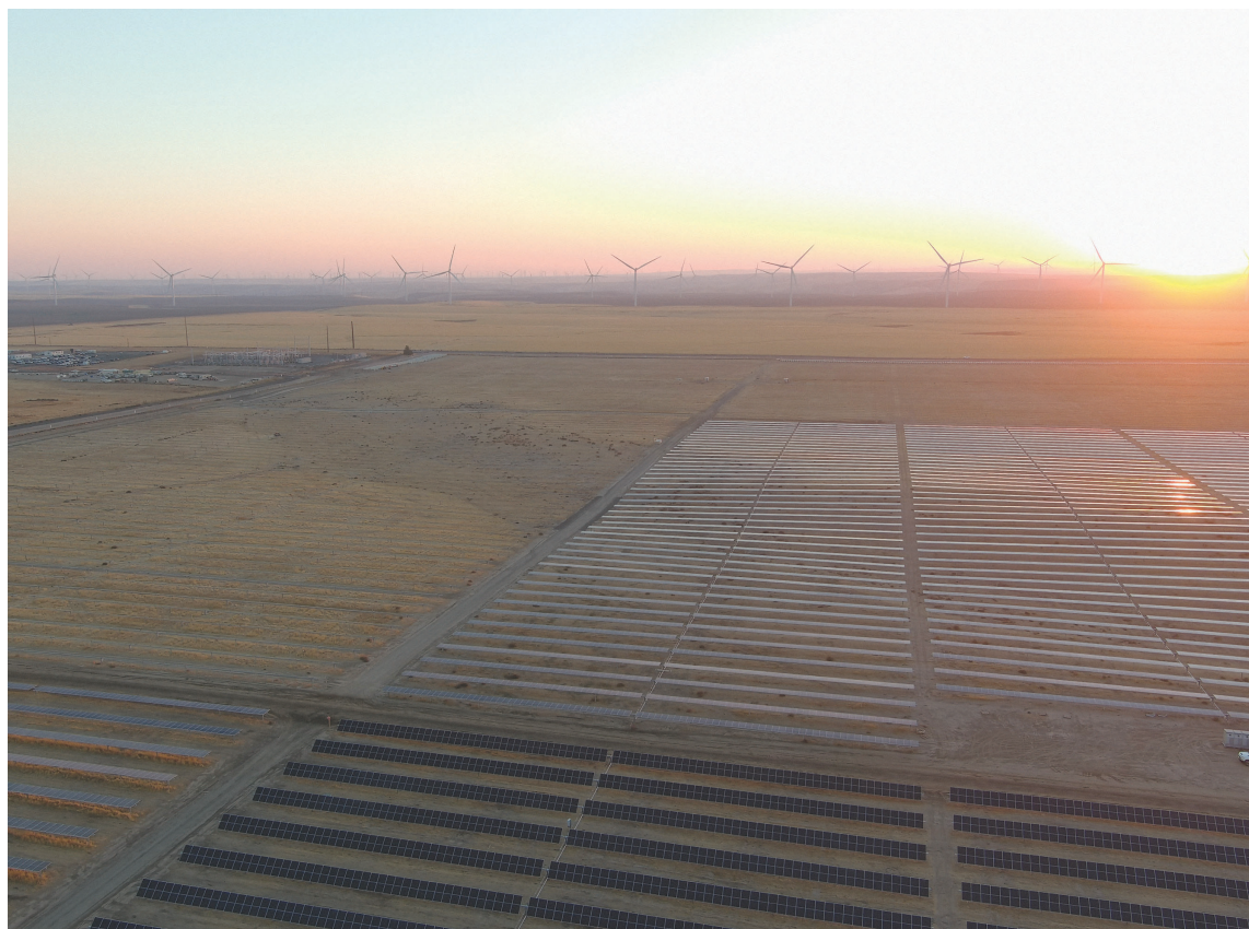
Avangrid Construction with Wind (image provided by Avangrid)
