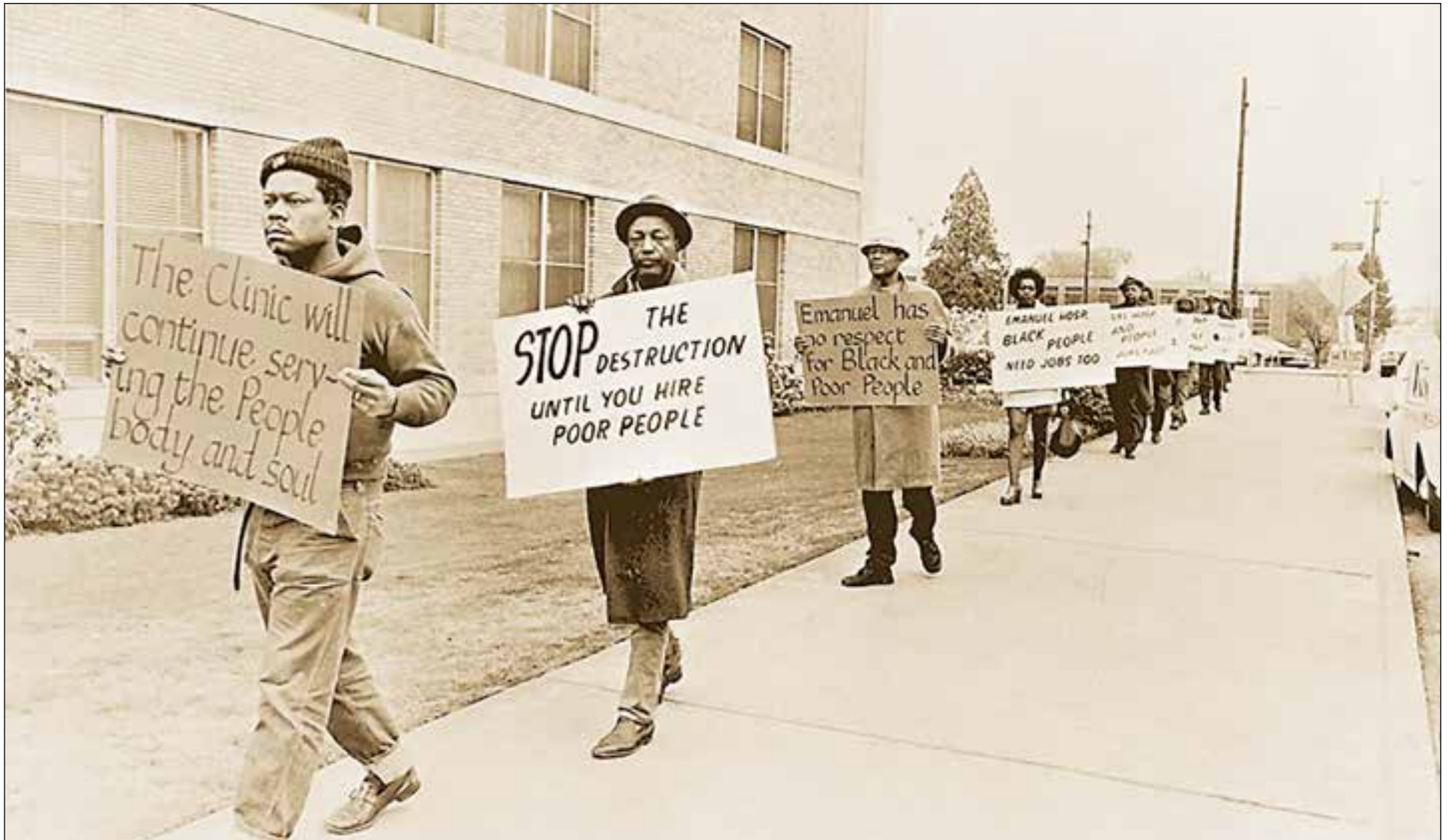
Black residents protest the forced demolition of neighborhood homes to make room for urban redevelopment and the expansion of Emanuel Hospital in north Portland in 1973. Nearly 50 years later, a new effort calls for the city to make restitution to Black families who were impacted. (Photo from Oregon Historical Society collection)
